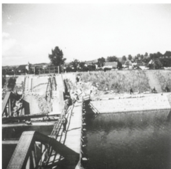
A4077-045-Brücke von Came
